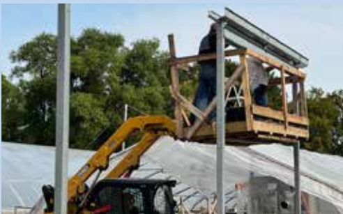
Ken and Gerald constructing.
